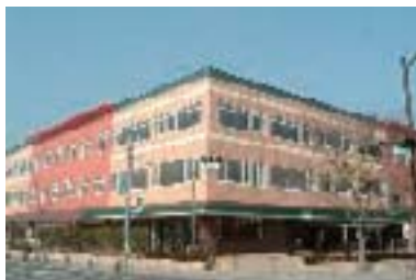
"i-Forest" information-related office building in Saga Prefecture
