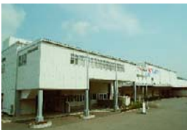
Warehouse of Hitachi Transport System, Ltd. used for customer distribution operations
